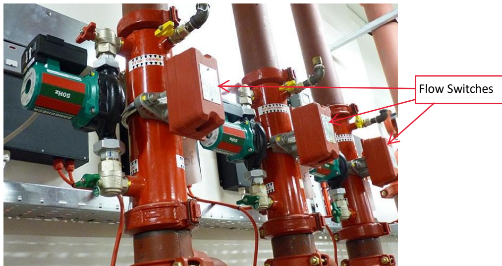
Typical sprinkler system header showing sprinkler system risers with three water flow switches
