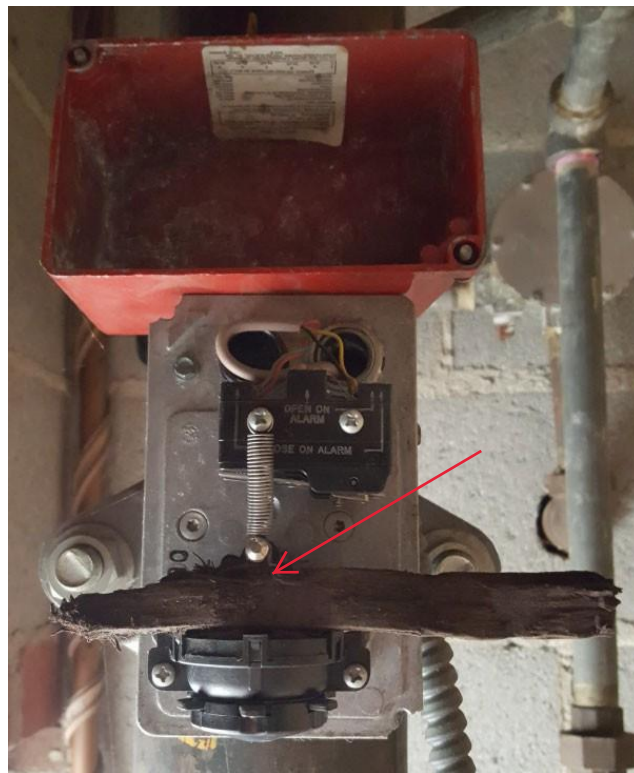
Picture above shows a piece of wood lodged preventing the paddle from moving
