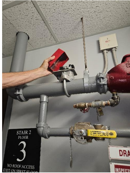
Removing Switch Cover
