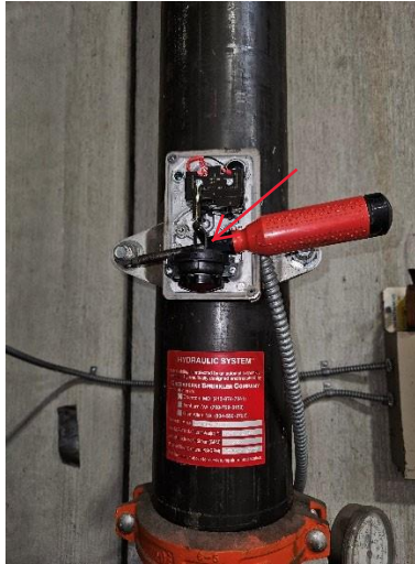
Screw driver to wedge the stem
