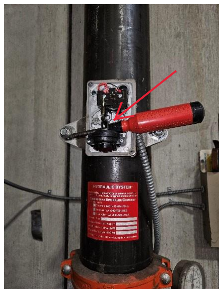
Screw driver to wedge the stem
