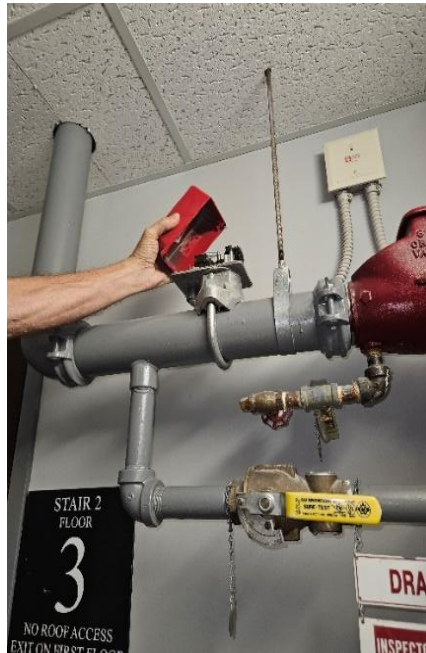
Removing Switch Cover
