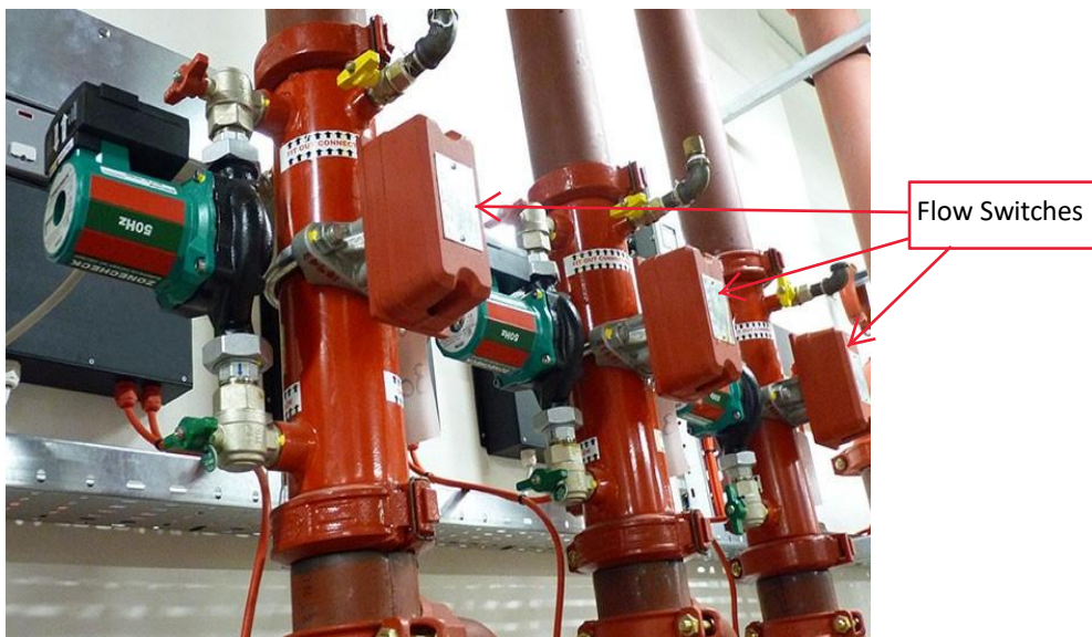
Typical sprinkler system header showing sprinkler system risers with three water flow switches.
